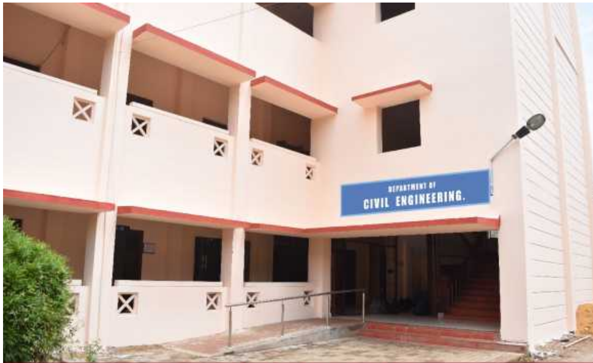
CIVIL ENGINEERING BLOCK
