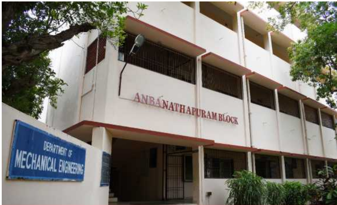
MECHANICAL ENGINEERING BLOCK
